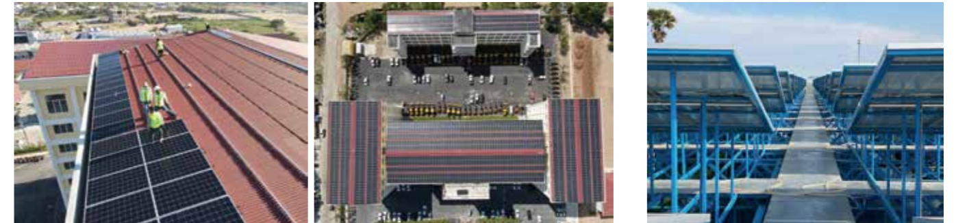
Cambodia 800KW Ongrid Project
